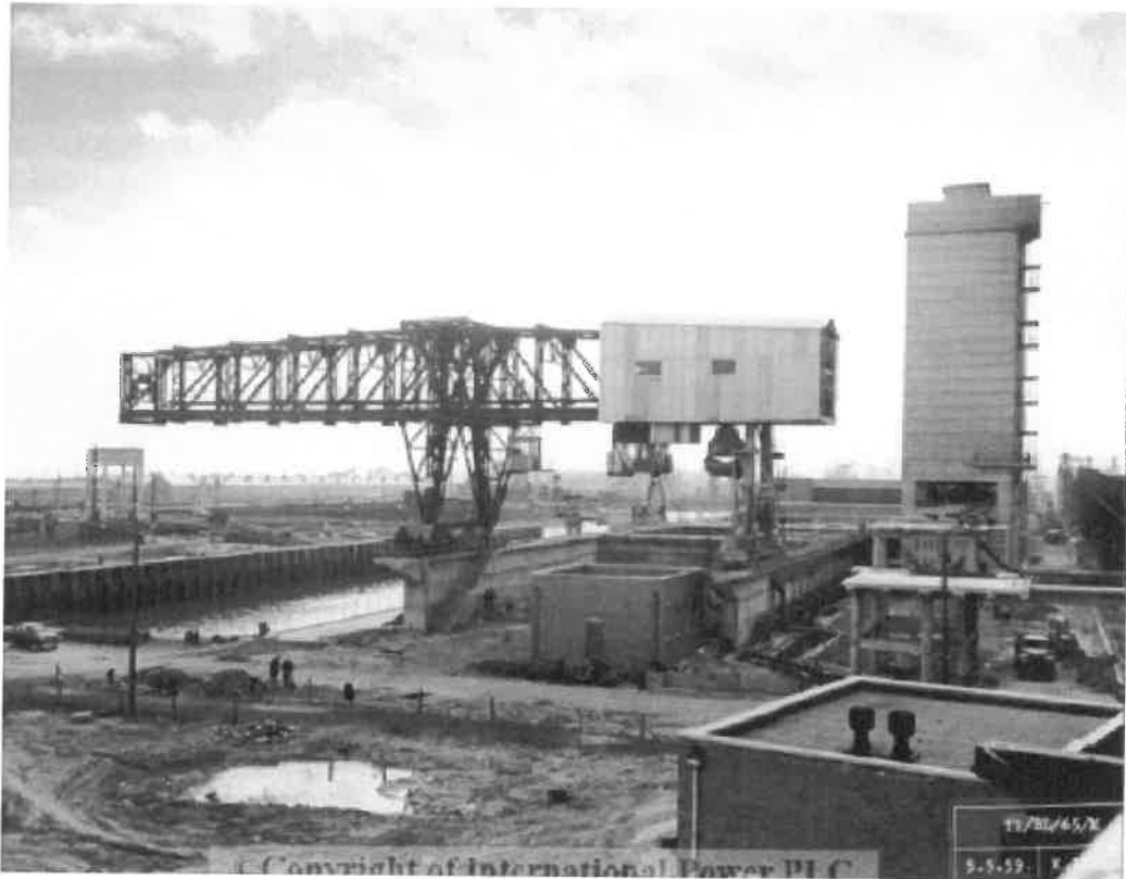
Figure 6. Ash Dock Under construction
