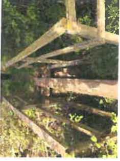
C Bridge over drainage ditch
