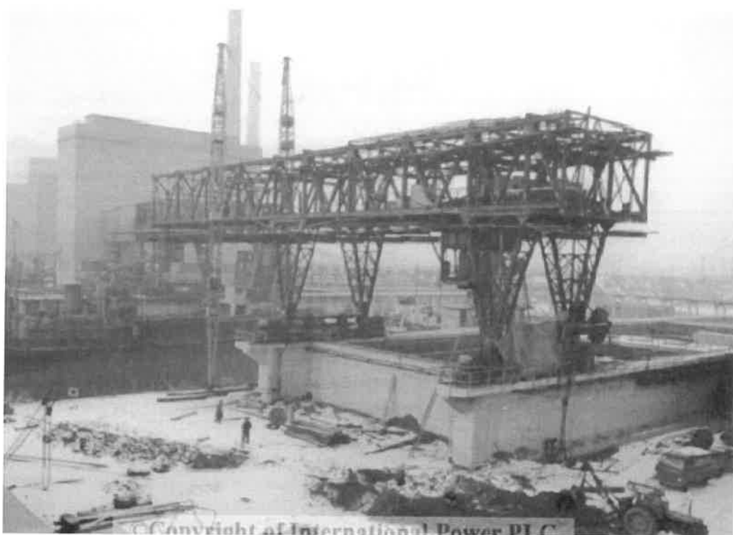
Figure 7. Ash Dock under construction
